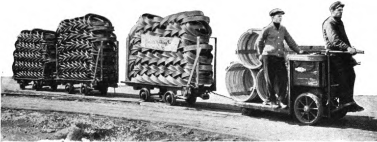
Industrial Electric Trucks are an economic factor widely adopted for transporting freight and baggage in railway and steamship service. In and around manufacturing plants they are used extensively for delivering loads where electric cranes are not practical.
